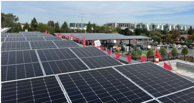
Solar rooftop (left) and carport (right) PV arrays located at the Belle Haven Community Campus.
