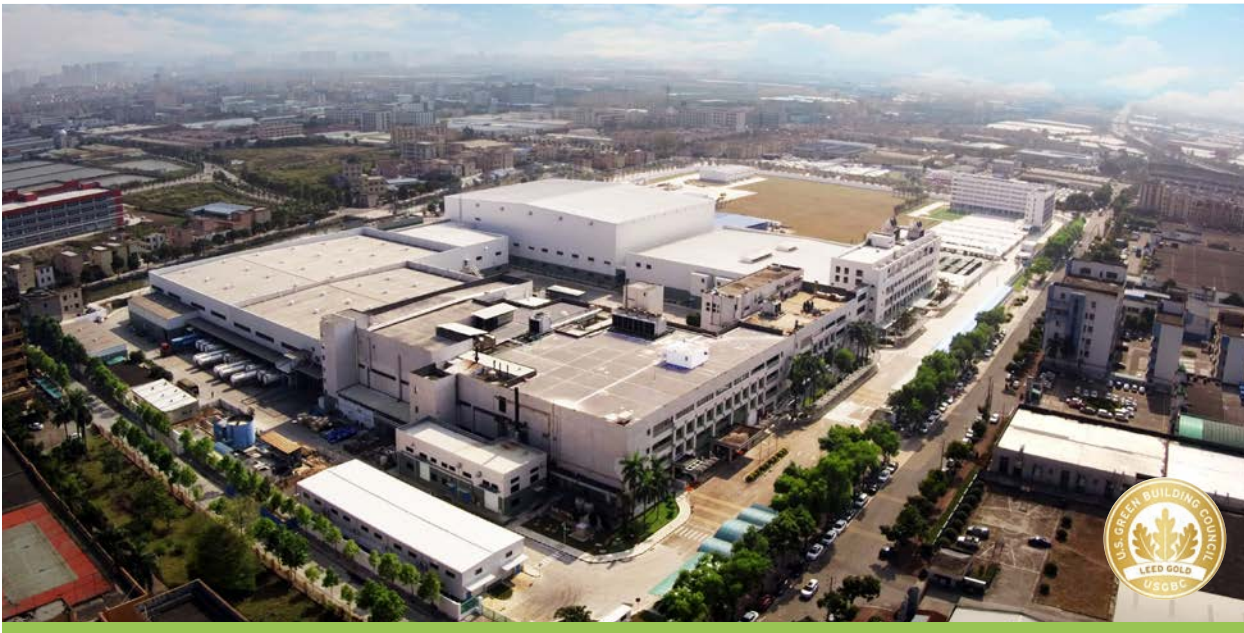
Colgate, Hawley & Hazel Oral Care manufacturing facility in China.
